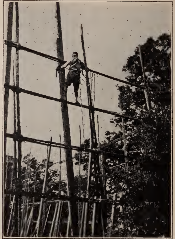
ERECTING THE SCAFFOLDING FOR VORNHOLT MEMORIAL
